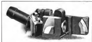
Fig. 3176. Sewall Steam Coupler, No. 20 AF.
